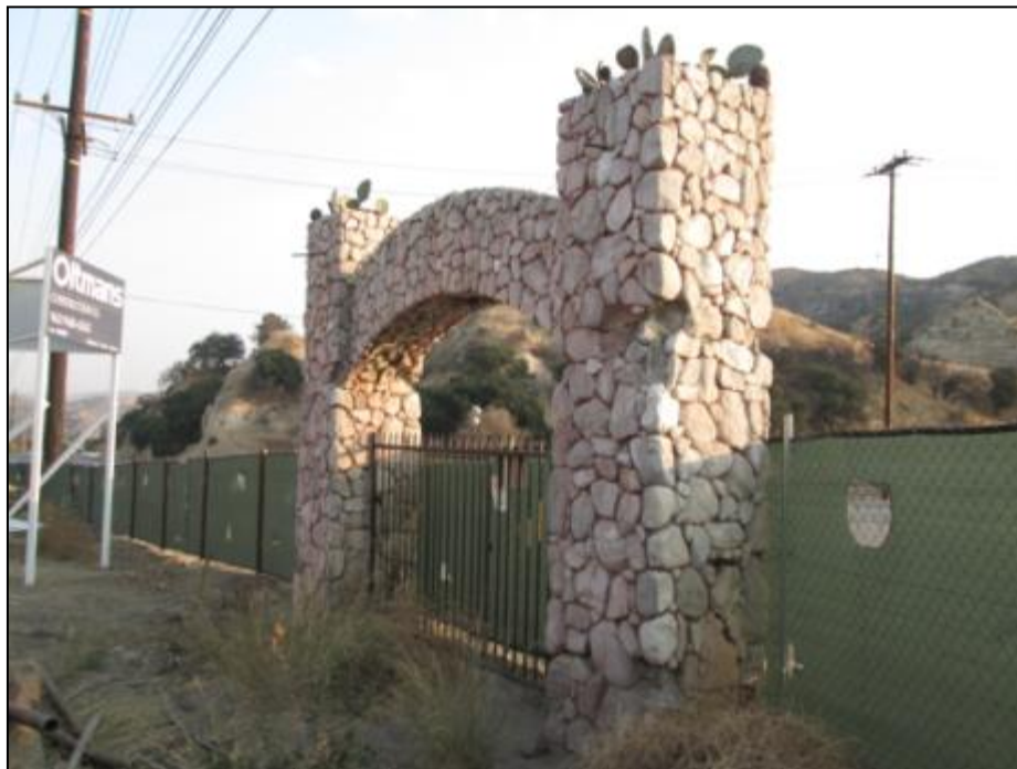
West façade of the Live Oak Manor arch. View looking northeast.
