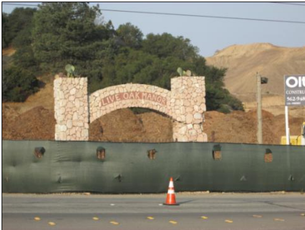
Live Oak Manor stone arch within construction site for Gate-King Project on Sierra Highway. View looking west.
