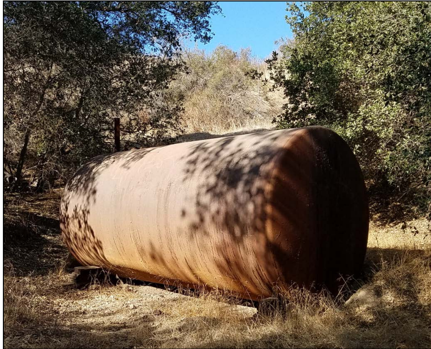
6,000 gallon water tank constructed of steel plates riveted and welded together. View looking west.
