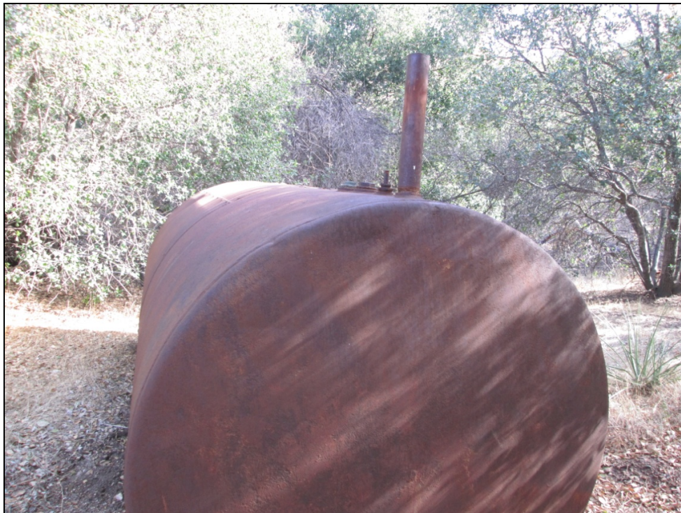
West end of tank with the intake pipe extending from the top of the tank. It appears that the tank was filled by a gravity fed water conveyance system gathering water from the local springs, or a small naturally fed reservoir.
