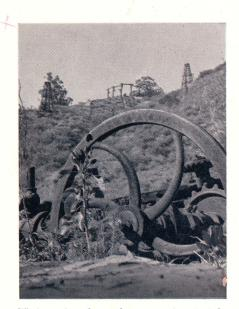
The remains of an old steam engine. At left, the cylinder, flywheel and sprocket. This may have been used to drill No. 4
