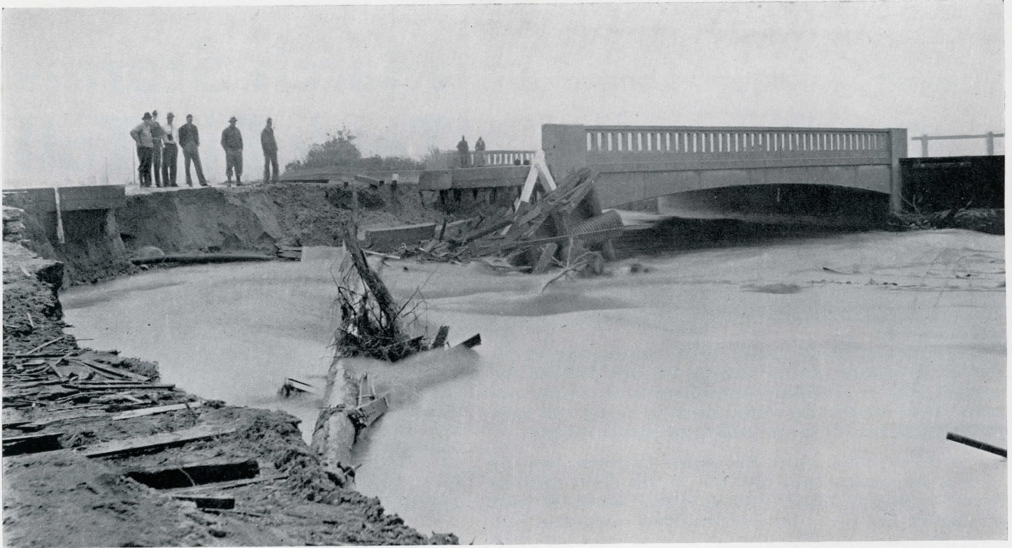
High waters in Barton Wash ripped away timber wing on this bridge on Route 168-C in Los Angeles County.
